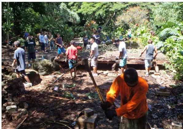
Hi'ipaka staff and volunteers restore the amphitheater in the back of the valley. It took nearly four months of Saturdays to complete. - Photo: Waimea Valley Hi'ipaka LLC
