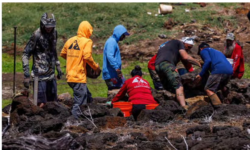
The Kānei'olouma restoration project is currently centered on two preservation efforts - clearing decades of debris from its ancient fishponds and restoring its interior walls. In these photos, 20 young apprentices are being trained in the ancient art of uhaū humu pōhaku (dry stack masonry) by master stone masons such as Peleke Flores.
