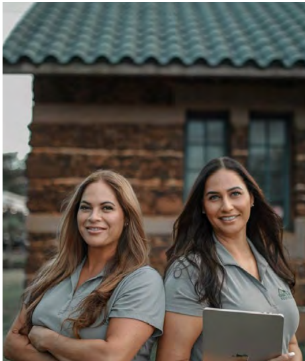
Lana Simmons (left) and Alia Galvez (right) standing in front of their finished roof at the historical Kaua'i Museum. - Photo: Charlie Valentine
