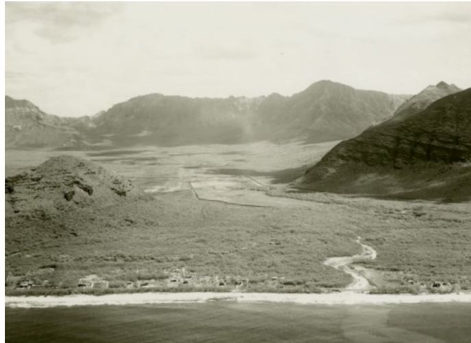
An aerial view of the PVT site area in Nānākuli circa 1930. - Photo: Courtesy of 'A'ole PVT Landfill
