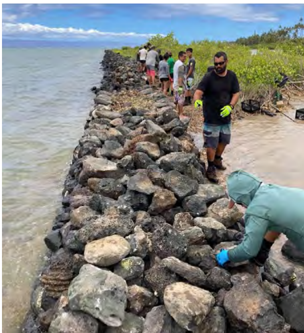
Volunteers help to repair a portion of the kuapā (fishpond wall) in 2021. The fishpond has three mākāhā (sluice gates) and its wall is more than 2,200 feet long.
