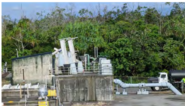
The first phase of repairs at the Hilo wastewater treatment plant includes replacing the "headworks" (where wastewater enters the treatment plant) which are deemed beyond repair. - Photo: Denver Collingwood
