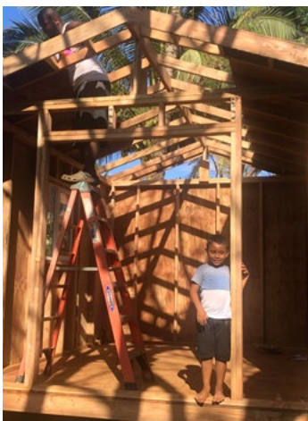
A self-quarantine unit going up. - Photos: Courtesy
