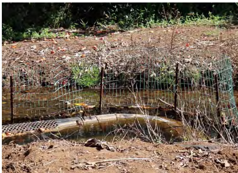
Breaks in the 'auwai causes pools of stagnant water and no flow to the lo'i. - Photo: Kawena Lei Carvalho-Mattos
