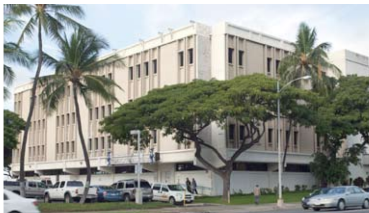
The Brownfields Assessment Grants will help assess contamination in six properties in Kaka'ako Makai, including the AAFES building, pictured. - KWO file photo
