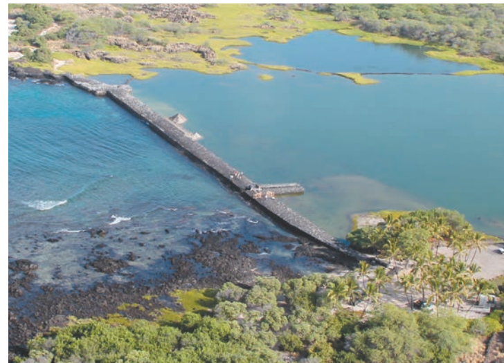
Aerial view of completed Kaloko kuapā at Kaloko-Honokōhau National Historical Park. - NPS photo by Adam Johnson
