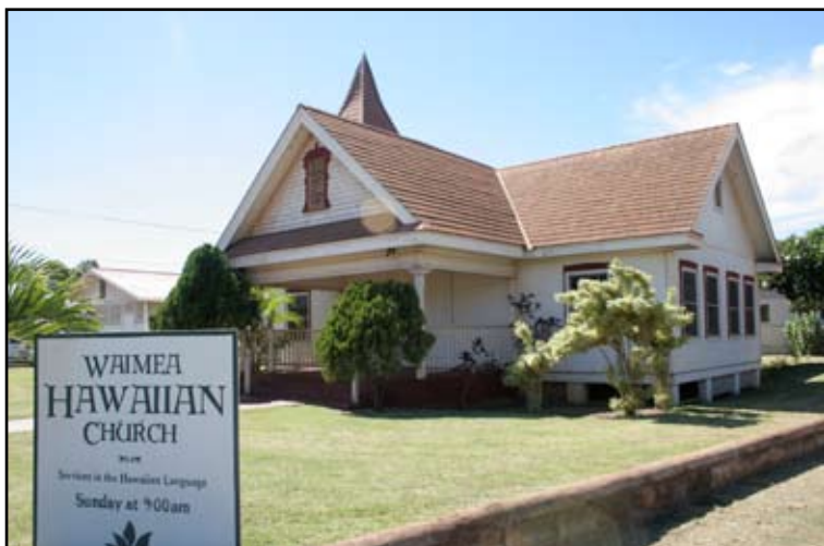
The land under the Waimea Hawaiian Church was among two parcels deeded to the 'Ohana Ni'ihau o Waimea Ekalesia to redress past wrongs. - Photo: Blaine Fejerstrom
