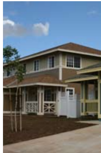
DHHL's 326-unit Kaupē'a project in Kapolei is nearly half-filled with native Hawaiian families. - Photo: Courtesy of DHHL
