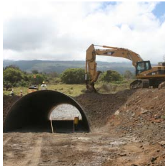
Infrastructure development at Kēōkea-Waiohuli Homestead. - Photo: Courtesy of DHHL
